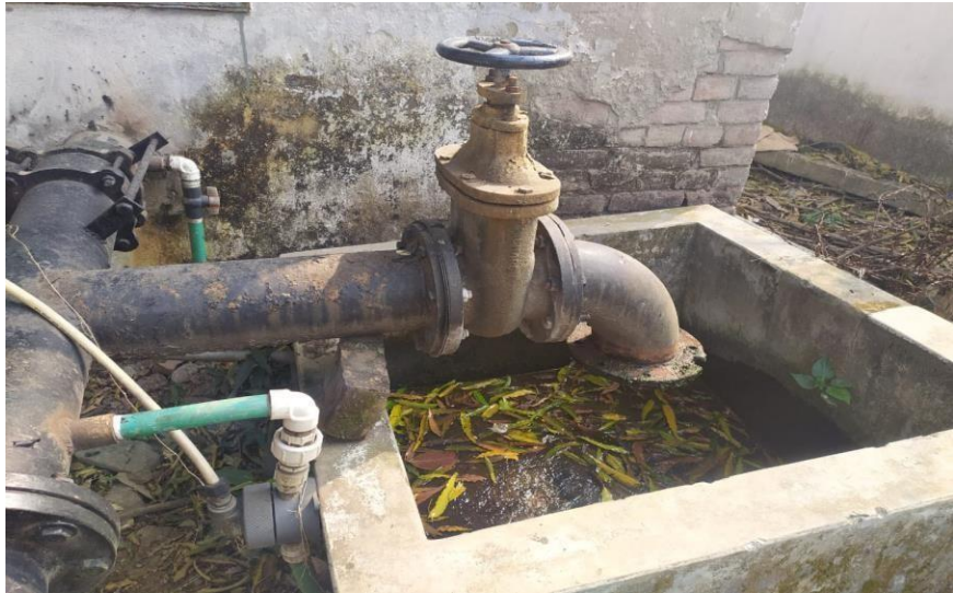
Figure 6. 10 Nazrul Islam Hall Pump Station
